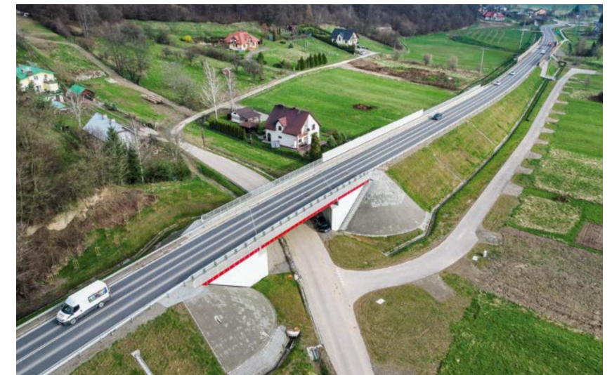
← Road No. III, Krtiny-Brezina Section, Czech Republic
